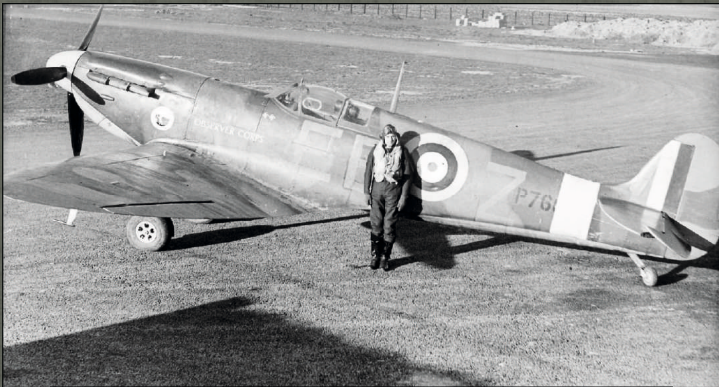
Spitfire Mk.IIa P7666 of No. 41 Squadron, RAF Hornchurch, late 1940. Well known photo of S/Ldr Donald O. Finlay in front of his personal Spitfire Mk.IIa, coded EB-Z. Note the blade shape of the Rotol RX5/1 constant speed propeller, the clearly visible on/off undercarriage indicator and highly polished aircraft surface. More about D.O.Finlay in colour profile B. (photo: Simon Erland)
