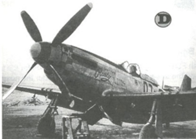
The Aeroproducts propeller used on the P-51K shows up clearly in this photo of Rusty taken in the snow in February or March 1945. Note the air breather plate, the uncowed exhausts and the bulged canopy.
