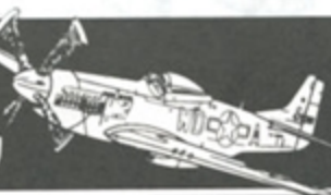
The Aeroproducts propeller used on the P-51K shows up clearly in this photo of Rusty taken in the snow in February or March 1945. Note the air breather plate, the uncowed exhausts and the bulged canopy.
